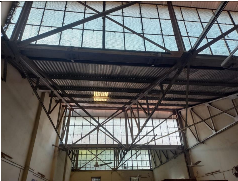
View of lattice girder and north light roof truss
