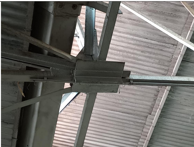
View of lattice girder and north light roof truss
